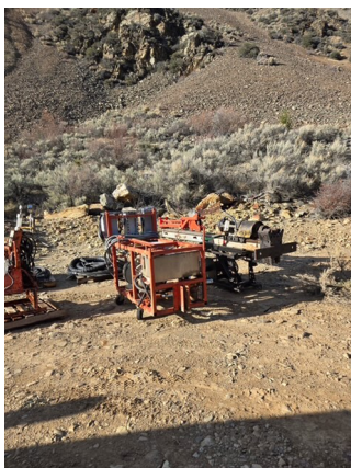
Diamond Drill Mobilized to site.
