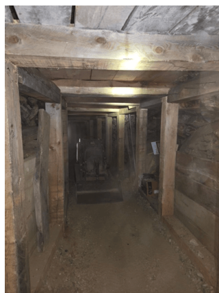
Zero Level – Rehabbing of the access drift
